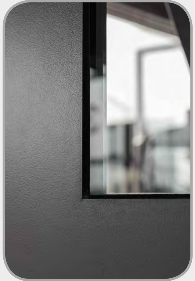
Glazing, flush on one side
