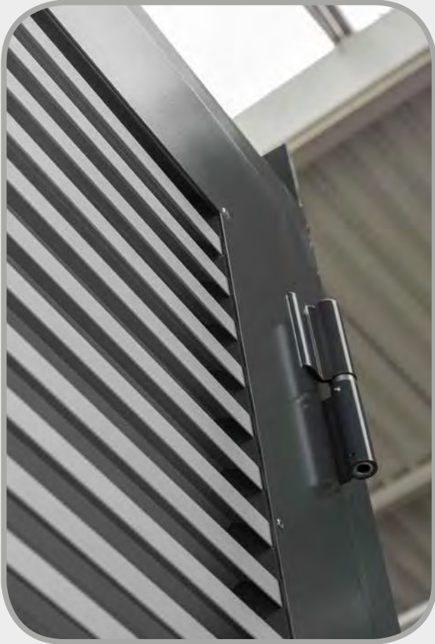
Ventilation grille, flush on one side
