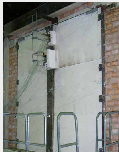
Fire test, MPA Braunschweig
